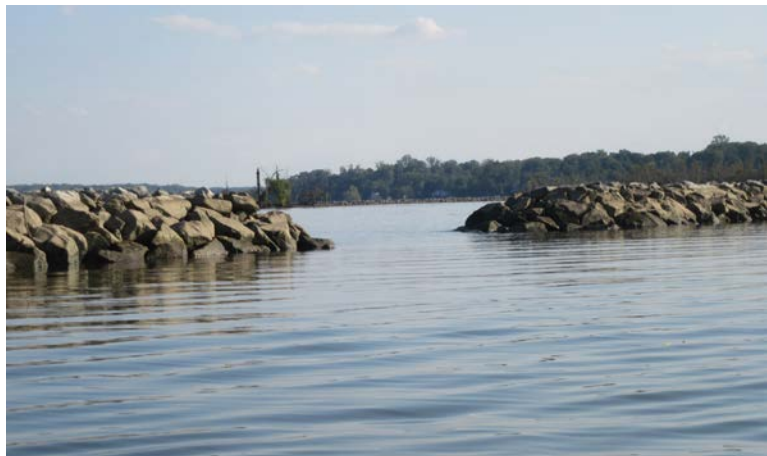
Rock sills built as part of the marsh stabilization project Photo by Glenda Booth
